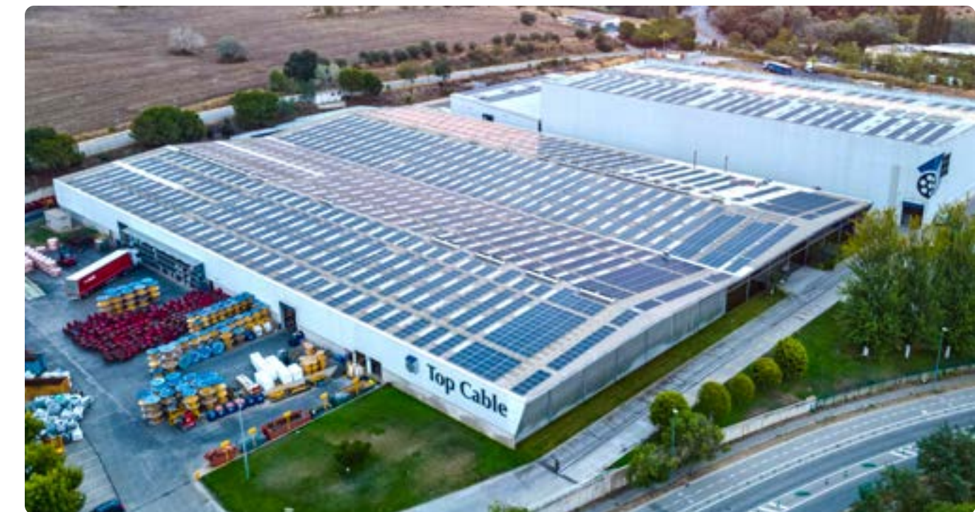
Rubí (Barcelona) headquarters has 6.492 panels (2,83 MW).
