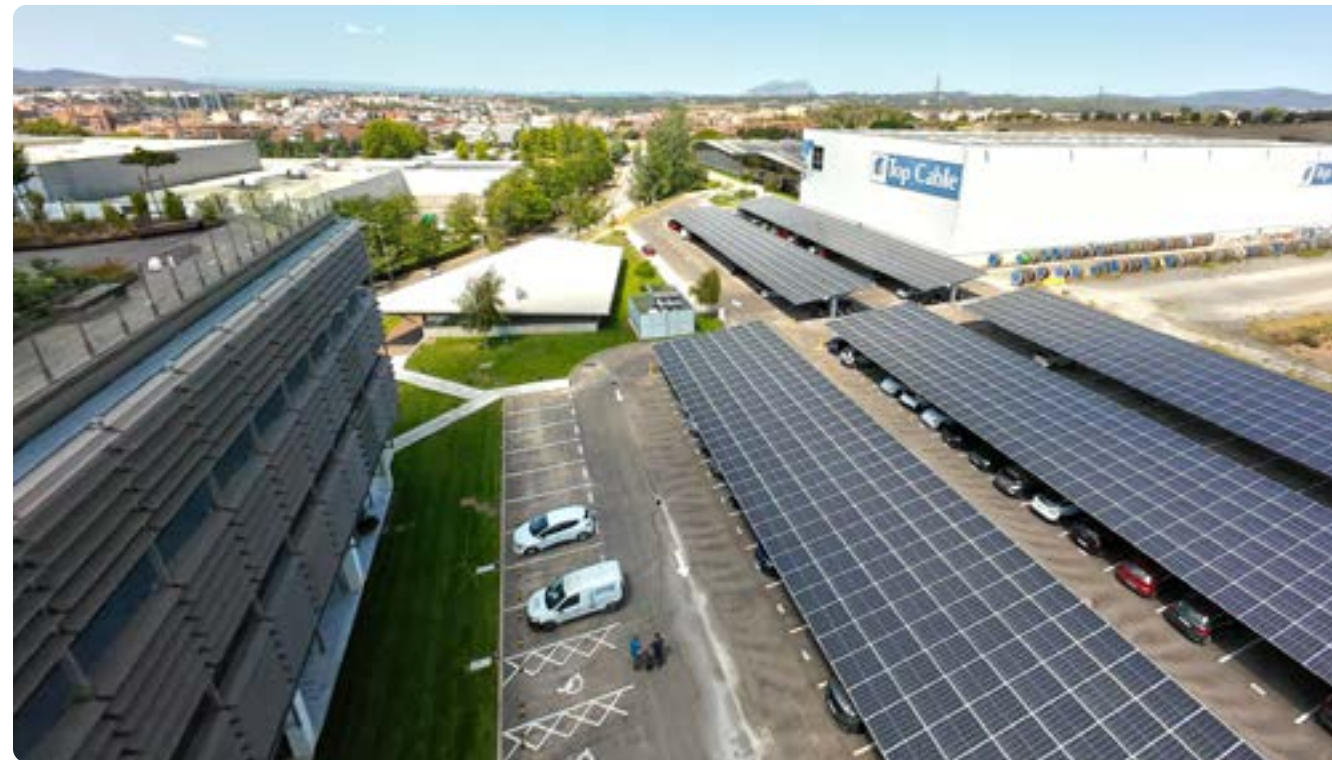
The recharging system includes 158 charging points with 7,2 kW individual power.
